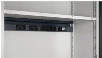
Raceway applied on the bottom part of the perforated shelf-panel
